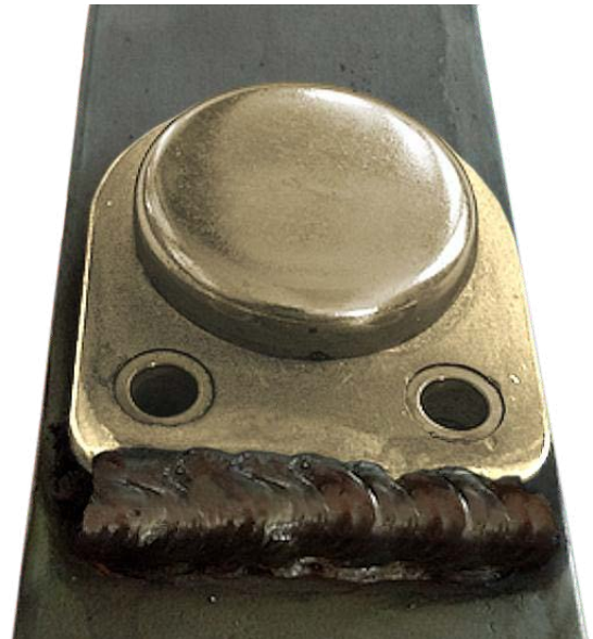
Correctly welded across the end of the tab
