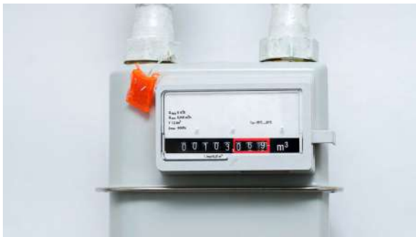
Maintenance of gas meters
