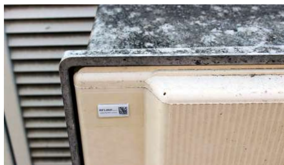
Inspection of electrical substations
